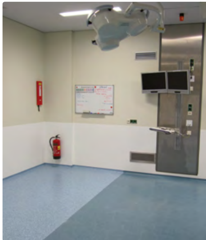
Project: Hospital operating theatres and other facilities | Installation: PALCLAD Pro HYG White with welding rods
