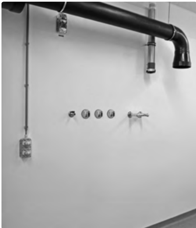
Project: Hospital operating theatres and other facilities | Installation: PALCLAD Pro HYG White with welding rods
