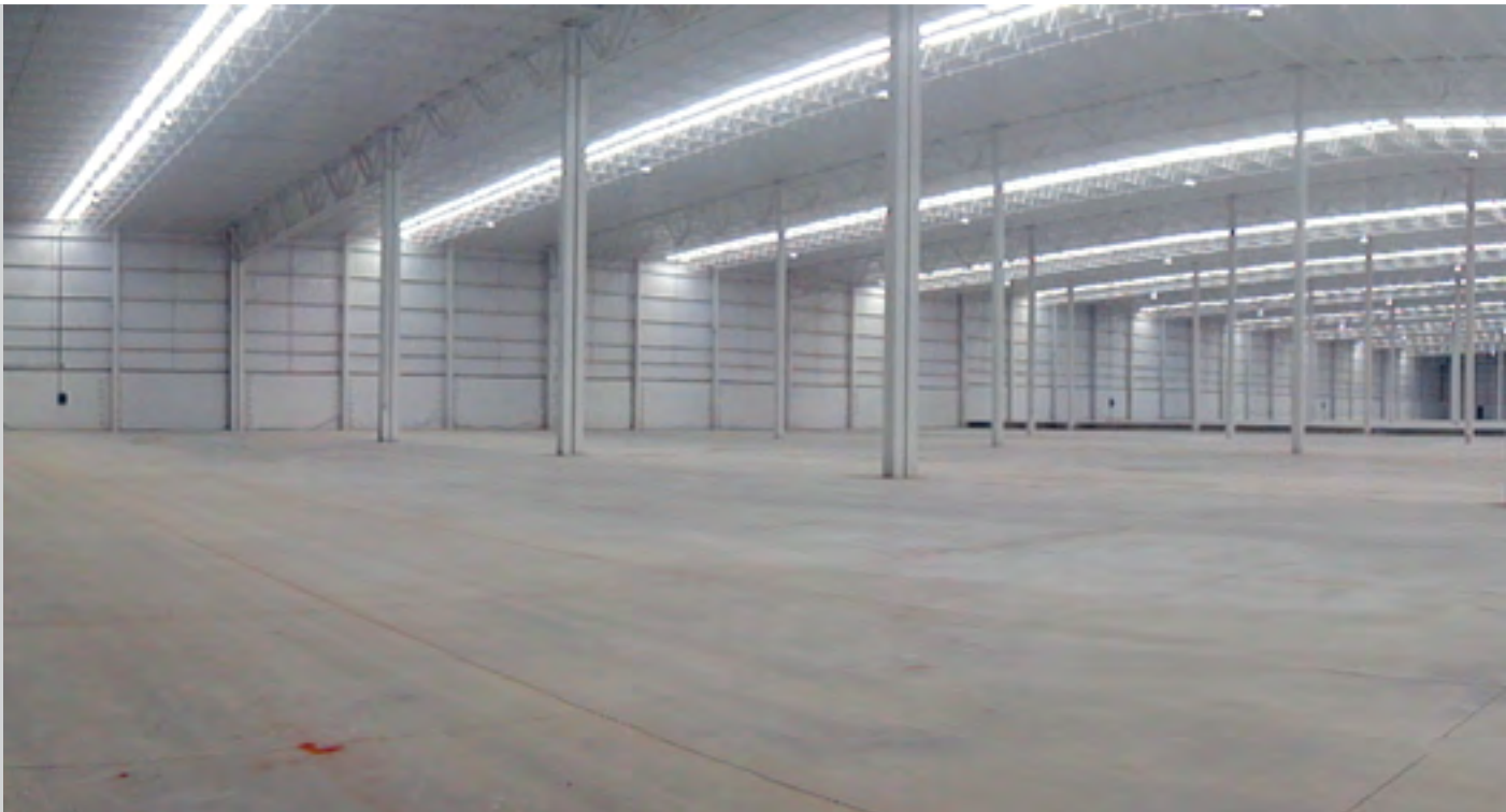
SUNTUF® Skylights Installed
