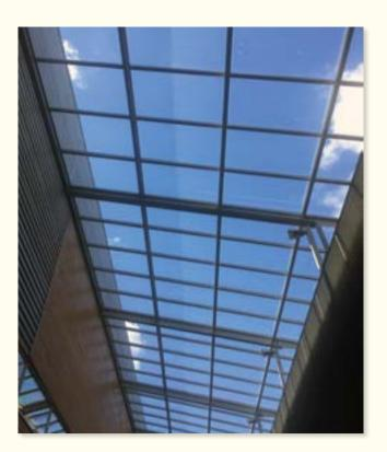
PALSUN<sup>®</sup> flat polycarbonate panels were chosen to replace glass in facades and canopies of shopping centers in Lithuania. Through our Lithuanian distributor Avisma, Palram matched the characteristics of the original glass panels and provided a solution that is more durable than glass, and is safer for the visitors to the shopping centers.
