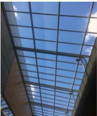
PALSUN® flat polycarbonate panels were chosen to replace glass in facades and canopies of shopping centers in Lithuania. Through our Lithuanian distributor **Avisma**, Palram matched the characteristics of the original glass panels and provided a solution that is more durable than glass, and is safer for the visitors to the shopping centers.
